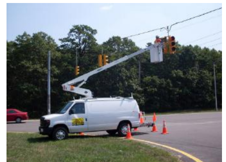
🔧 Traffic signal relamp at Town of Brookhaven intersection. Hinck is a leading traffic signal maintenance contractor on Long Island, currently maintaining over 1000 signals – 24 hours a day, 7 days a week.
